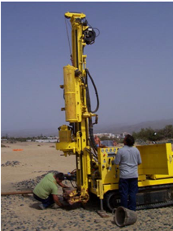
Fig. 2: Drilling vehicle on site ready to proceed with the drill process.
